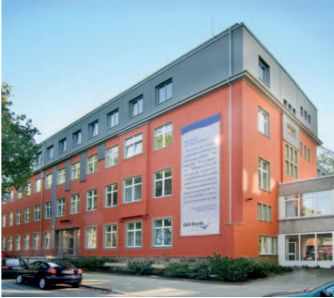
GLS Bank Headquarters in Bochum, Germany.
